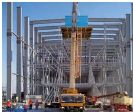
ULD System – New Doha International Airport
